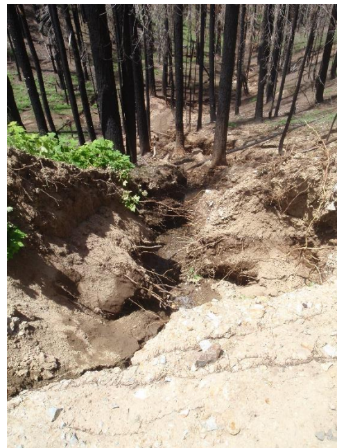
Figures 3A-B. Example of crossing (site H7) where plugged culvert failed resulted in flow diversion, in this case a long run along the roadway (3A) with gullying where flow finds a return path to the stream channel (3B).
