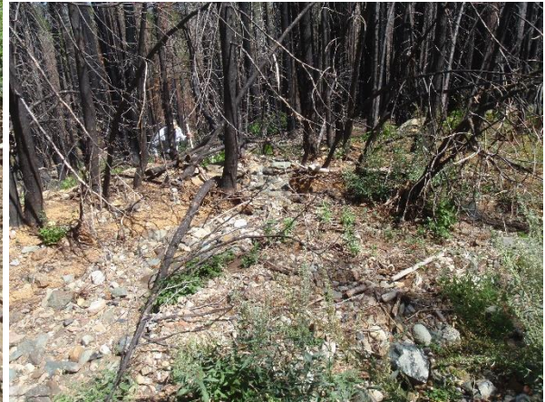
Figures 7A-B. Example of road surface erosion (7A) resulting from culvert failure and diversion of flow onto roadway. Erosion also occurs where flow leaves roadway and returns to channel, as shown in Figure 7B. Site is LG 33 on FS road 24N08X.
