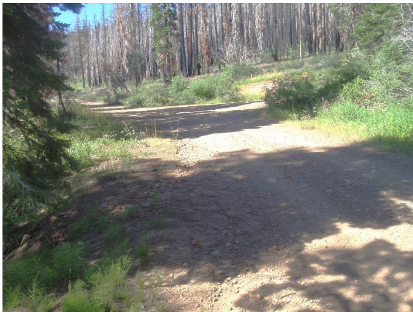
Figures 8 and 9. Examples of surface rilling from Hungry Creek Subwatershed (Site H11, Road 27N09) and Little Grizzly Creek (Site 56, Road 24N09).
