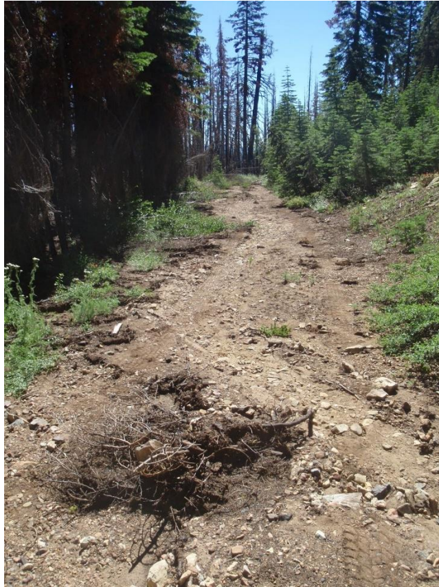
Figures 7A-B. Example of road surface erosion (7A) resulting from culvert failure and diversion of flow onto roadway. Erosion also occurs where flow leaves roadway and returns to channel, as shown in Figure 7B. Site is LG 33 on FS road 24N08X.
