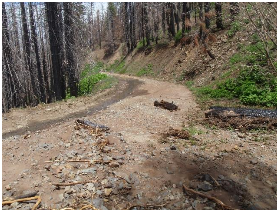
Figures 3A-B. Example of crossing (site H7) where plugged culvert failed resulted in flow diversion, in this case a long run along the roadway (3A) with gullying where flow finds a return path to the stream channel (3B).
